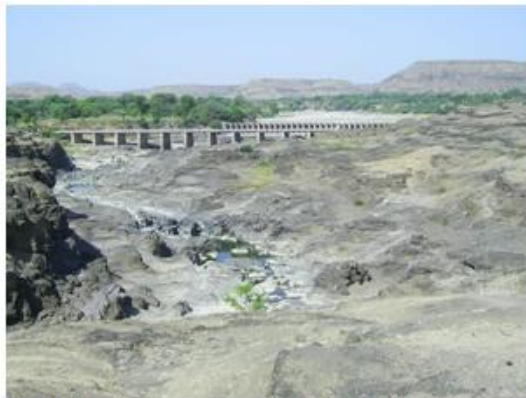
Photo 4 - An upstream view from the Mandwe Knick
