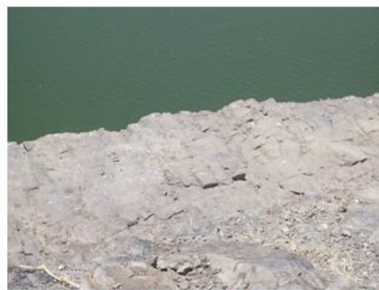
Photo 7 columnar basalts on the eroded section of bank wall
